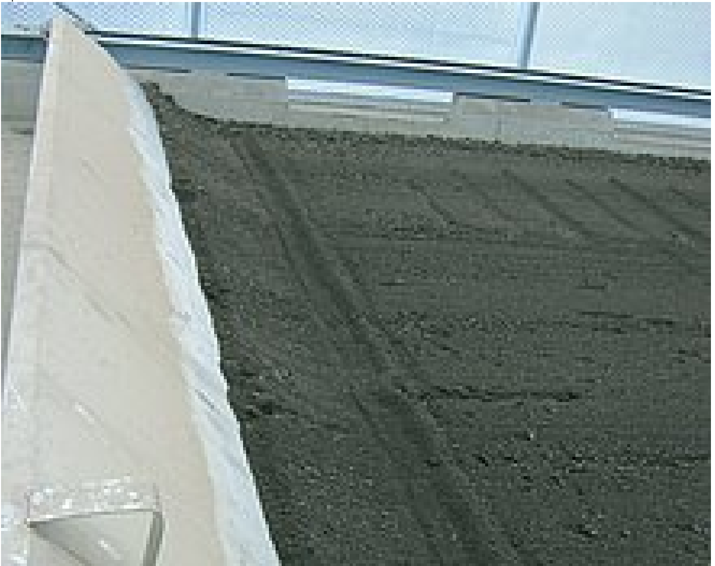
The dry sludge that lies a the half-pipe that is either taken out of the system or can be used for backmixing.
