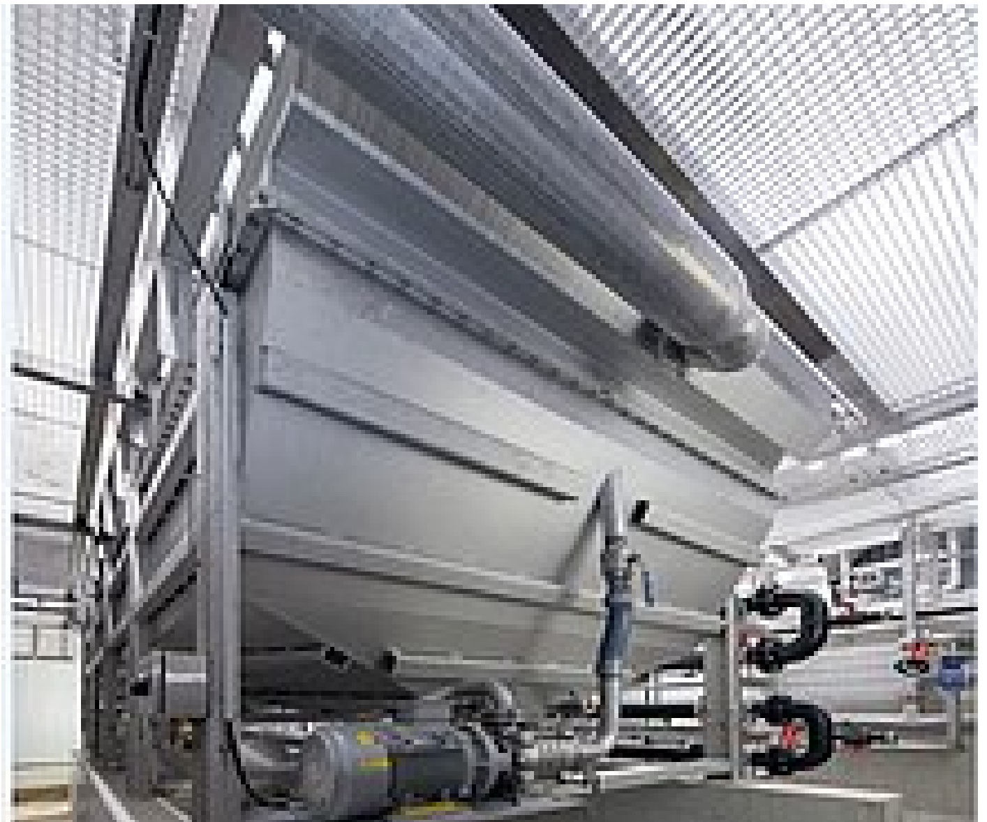
Fig. 3: HUBER Dissolved Air Flotation Plant HDF S 20
