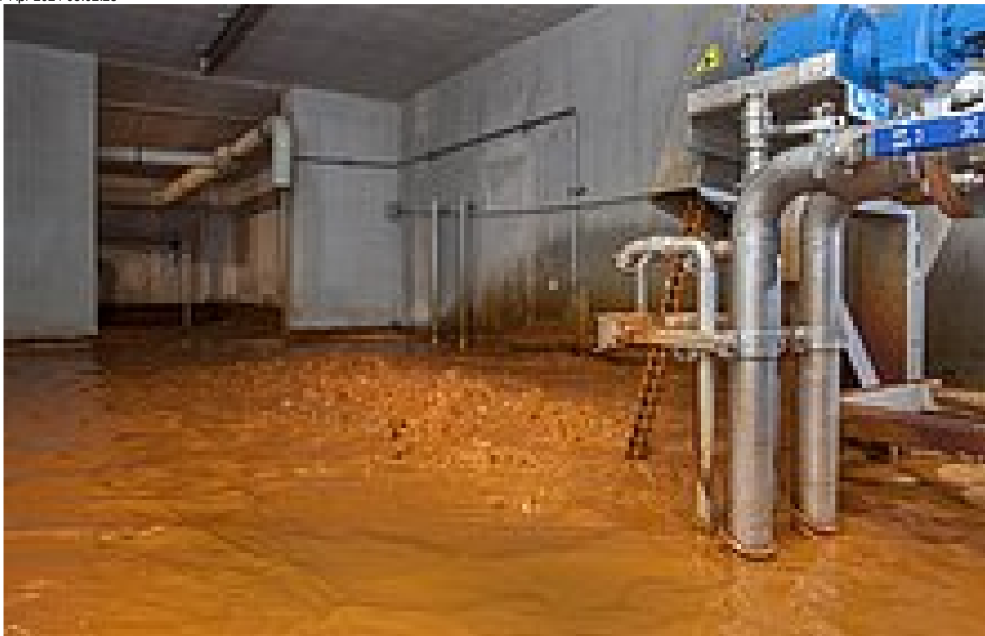
Fig. 4: MBR plant with a HUBER Membrane Filtration VRM@ 30/18 RF in one filtration chamber
