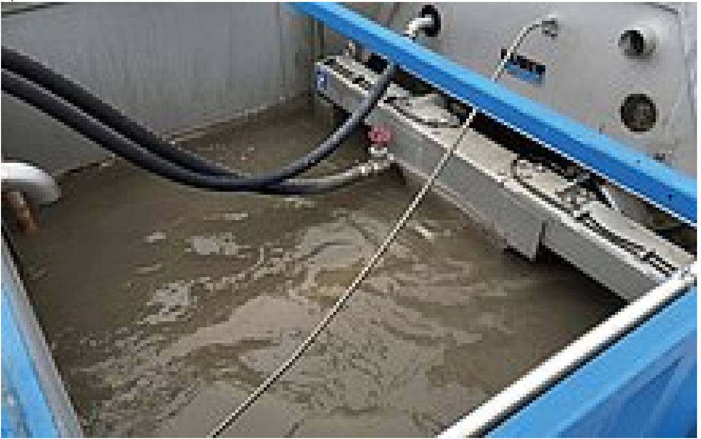
Flow to the HUBER Drum Screen LIQUID with maximum upstream water level
